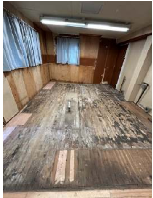
MRG kitchen stripped down in July.
