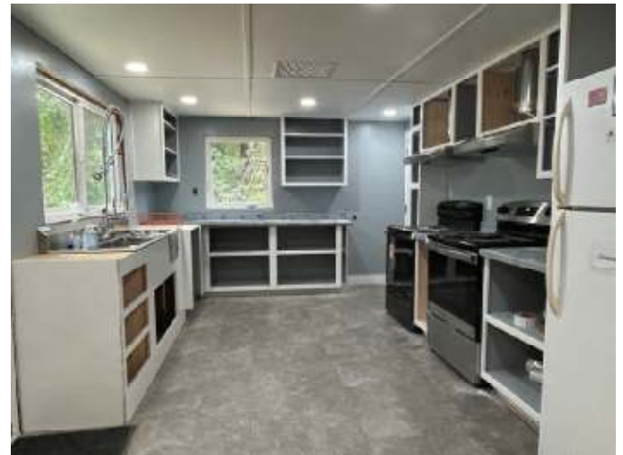
MRG kitchen remodel in progress in August.
