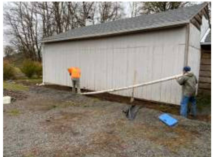
Kurt and Nate (along with Jim and Sonny) dug trenches and laid drainage for the gutters and water capture tank overflow around the MRG Junior Grange Hall, during wet weather.
